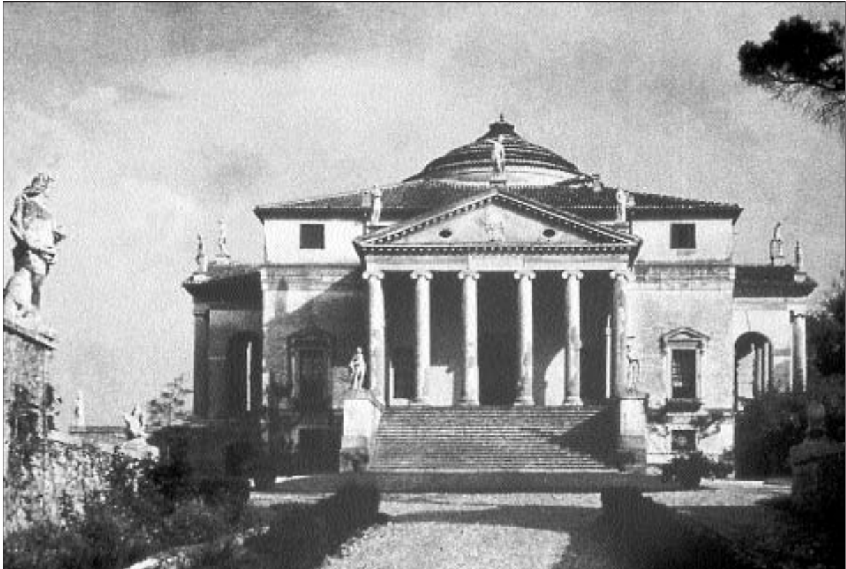
Fig. 8. NW façade of the Rotonda, view from the carriage approach.
