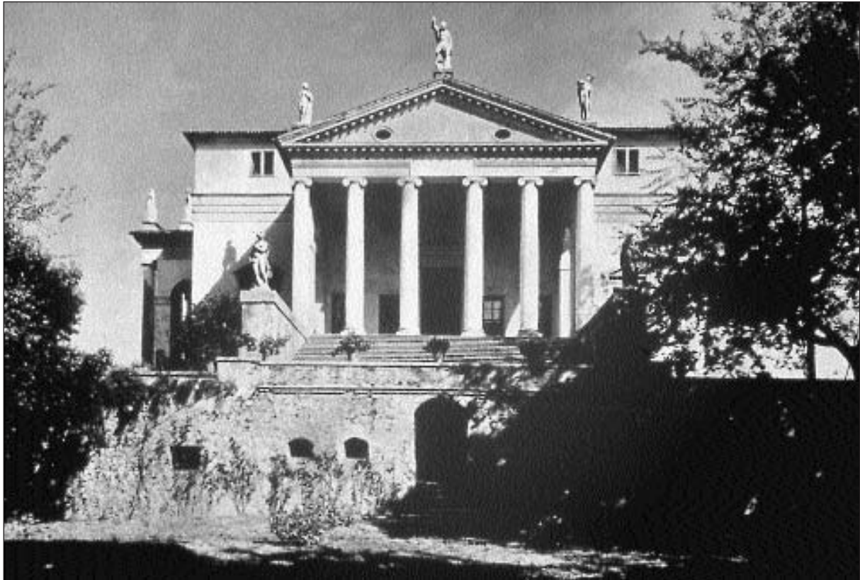
Fig. 10. SW façade of the Rotonda, view from the kitchen garden.
